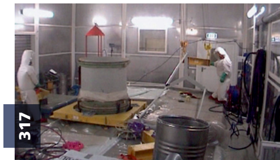
| Decommissioning activities at the Isotope Production in Rossendorf, Germany.
