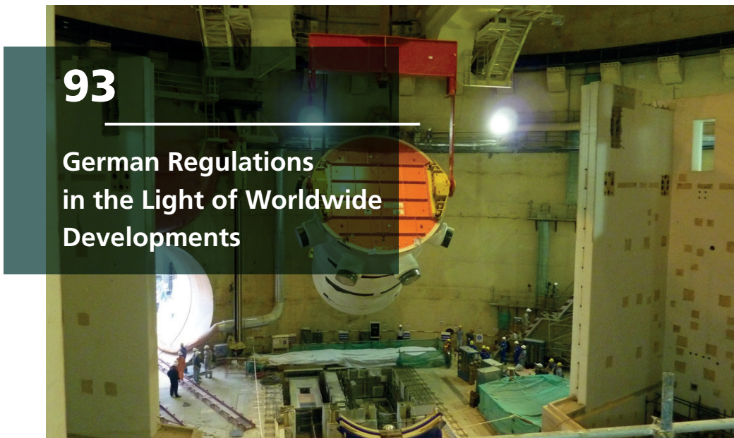
Installation of the reactor pressure vessel at the Tianwan nuclear power plant in China. (Courtesy: Taishan Nuclear Power Joint Venture Company (TNPJVC))
