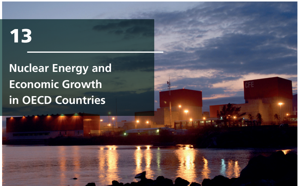
Aerial night-view of the Laguna Verde site in Mexico. Two boiling water reactors (BWR) with a gross capacity of 820 MWe each are in operation since the 1990s. (Courtesy: CFE)
