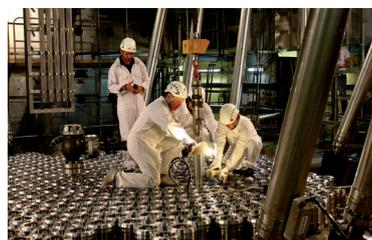
Positioning of the first fuel element into the reactor of *Atucha 2*. (Courtesy: NA SA)
